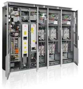
ACS880 multidrives with fieldbus adapters and feedback interface modules
